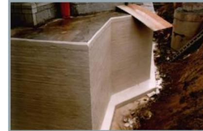
**Nitocote CM210** provides an excellent solution for waterproofing the outside or inside faces of basement walls and floors due to its ability to withstand both positive and negative water pressure. This makes it an ideal choice for waterproofing existing basements. The system is easily applied by brush, roller, trowel or spray and the completed solution gives both water, fire and CO<sub>2</sub> protection.
