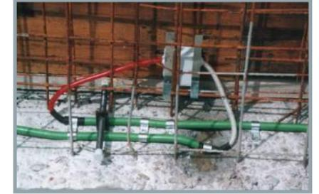
**Supercast Predimax** injection hose waterstops for future provision of sealing leaking joints.
