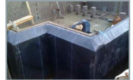
Post-applied bitumen based waterproofing for floors and walls can be easily installed using **Proofex GP / 3000** self-adhesive membranes in conjunction with **Proofex Protection Boards**. **Proofex 3000MR** is ideal where gas is present in the ground or the soil is contaminated. The aluminium foil layer in the membrane provides resistance and long term durability.
