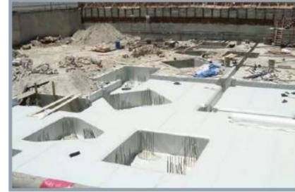
**Proofex PGP / Alkorplan**, a loose-laid PVC membrane system, is available in large rolls. Joining is realised through welding with hot air. Compartments can be laid out using **Supercast PVC** waterstops which are welded to the membrane.
