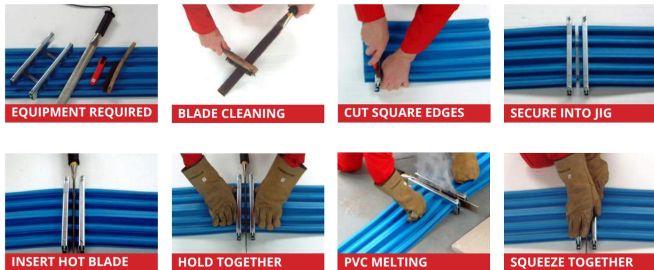
PVC waterstops should always be joined by welding using the process above, never by lapping. Fosroc supply jigs and heating blades suitable for making simple butt joints on site.
