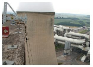
External refurbishment was required to five of the eight steelreinforced concrete cooling towers. The towers are 118m tall, with a base diameter of 95m, 45m at the top and 37m at the neck. The 40-year-old structures required a repair mortar that could protect from further carbonation and could be applied in thicknesses in excess of 50mm. The material needed to be lightweight due to the difficult application conditions. **Nitoprime Zincrich:** galvanic protection for exposed reinforcing steel
