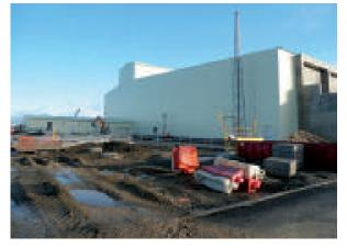
The construction of a convertor station on Deeside was required as part of the £560m interconnector project, designed to link the Irish and UK electricity grids. The contractor faced issues of ground subsidence, gas contamination and water ingress associated with high tides. Fosroc provided a solution encompassing water and gas proofing, joint sealing and concrete repair.
