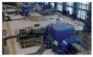
Fosroc supplied the new floor for the aluminium smelter power station at Fort William, as part of a major five turbine generator refurbishment. A durable and cost effective solution was required for replacing the uneven existing floor after the old turbines were removed. **Cemtop XD:** heavy duty, highly abrasion resistant selflevelling screed.
