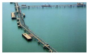
At South Hook, as part of the repair and strengthening of existing jetty and mooring structures, a cathodic protection system was installed. A compatible, sulphate resistant, cementitious material was required to cover a surface area of 14,000m<sup>2</sup>, at a thickness of 25mm. Fosroc's dry-spray concrete repair system **Renderoc DS** was used as a template for developing a material specifically for this project.
