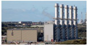
With a total generating capacity of 2,160MW and thermal efficiency of 60%, the Pembroke Power Station is one of the largest and most efficient CCGT power plants in the UK. The new natural gas fuelled compact industrial plant was constructed on a site formerly occupied by an oil-fired power station. Fosroc products were supplied over a 3 year construction period to different areas of the project:
